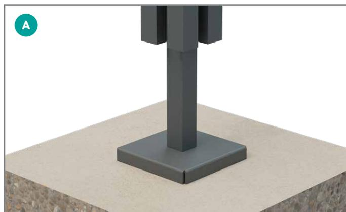
Then using a 4mm drill bit and a cordless drill, drill a pilot hole through the drill line in the front centre of the post for the self-drilling screws 50mm above the base plate and then at 100mm centres going up the post. Ensure you have a minimum of 4 fixings per post and the screws are in the centre of the channel.
