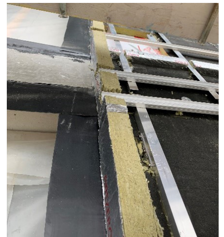
Figure 5: Typical installation of vertical cavity barrier (work in progress)
