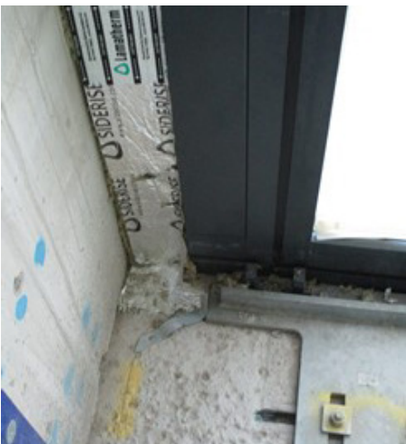
Figure 3: Typical vertical fire-stop with smoke foil
