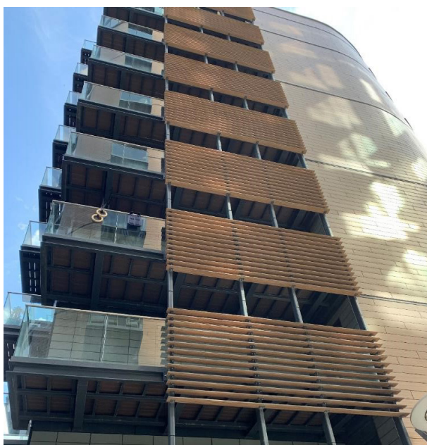
Figure 23: Balconies with timber decking and timber brise soleil
