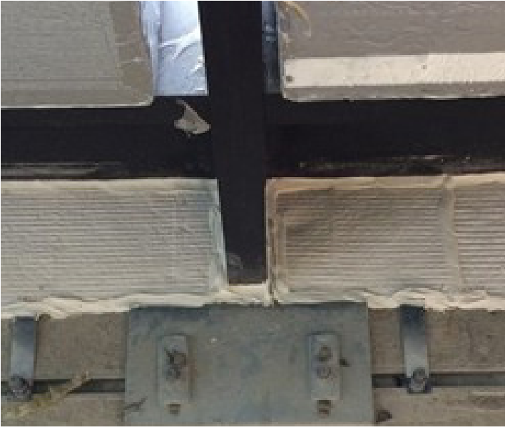
Figure 1: Typical horizontal fire-stopping with ablative coating
