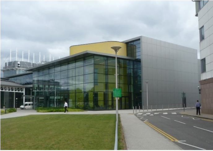
Figure 15: Typical ACM cladding
