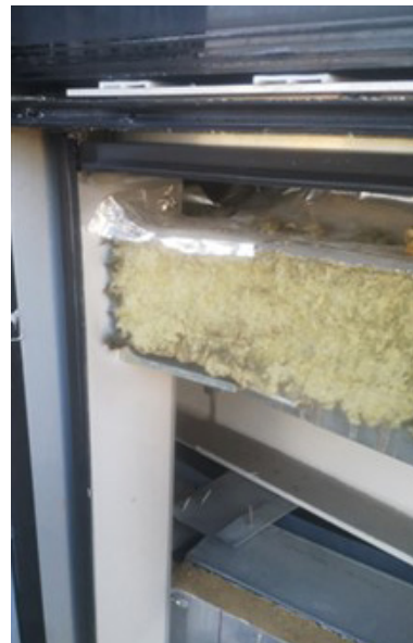
Figure 9: Typical fire-stop behind spandrel panel
