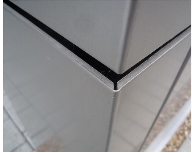
Figure 16: Close-up showing ACM core (seen at joint panel)
