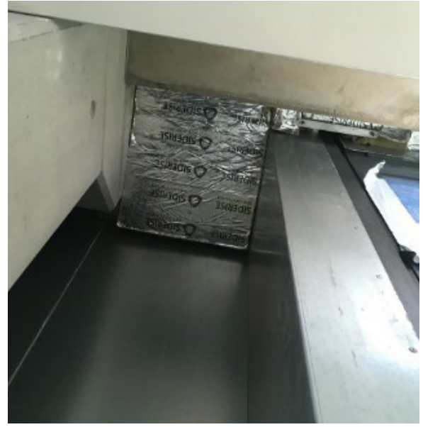
Figure 2: Typical horizontal fire-stops with smoke foil
