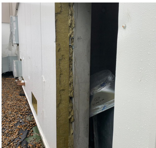
Figure 13: Typical metal insulated panels with mineral wool core
