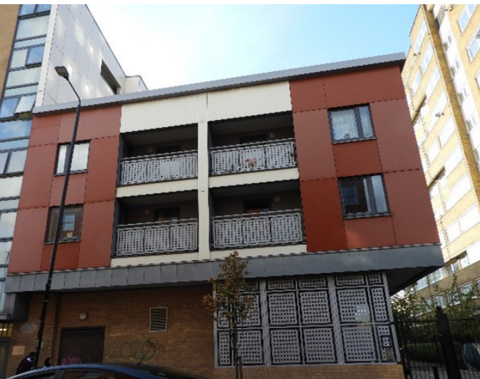
Figure 17: Housing block with HPL cladding
