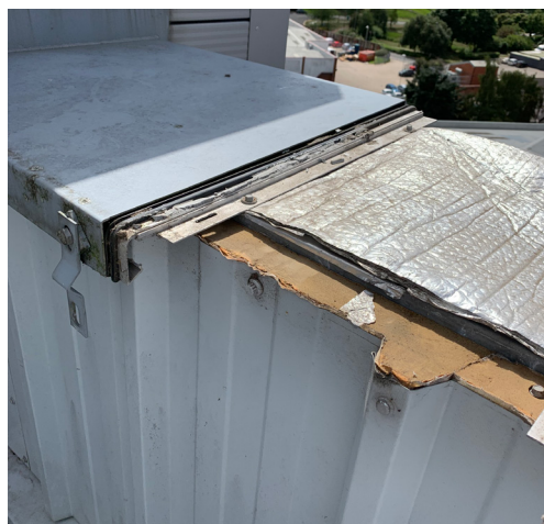
Figure 14: Typical metal insulated panels with PIR/PUR core
