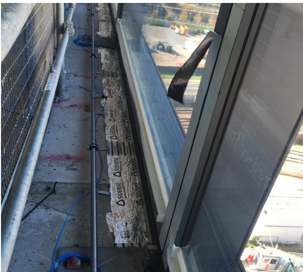
Figure 8: Typical installation of curtain walling and fire stopping
