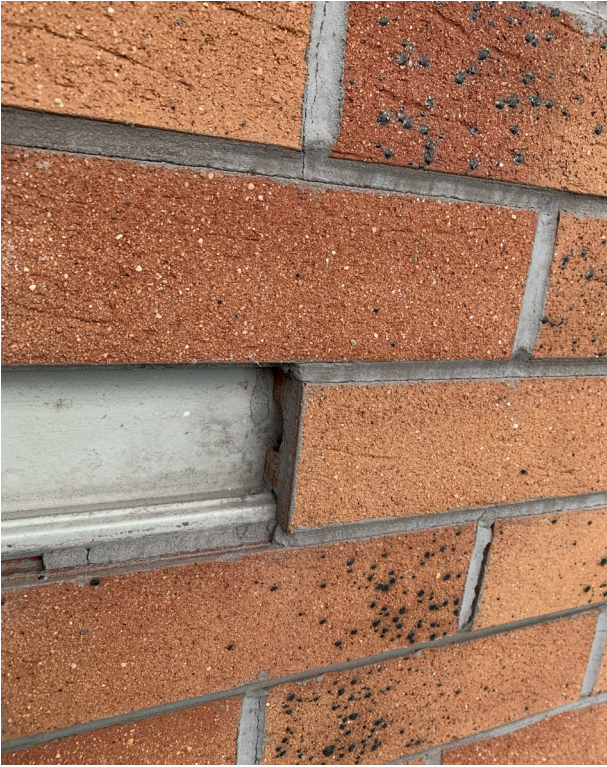
Figure 20: Close-up view of brick slip system
